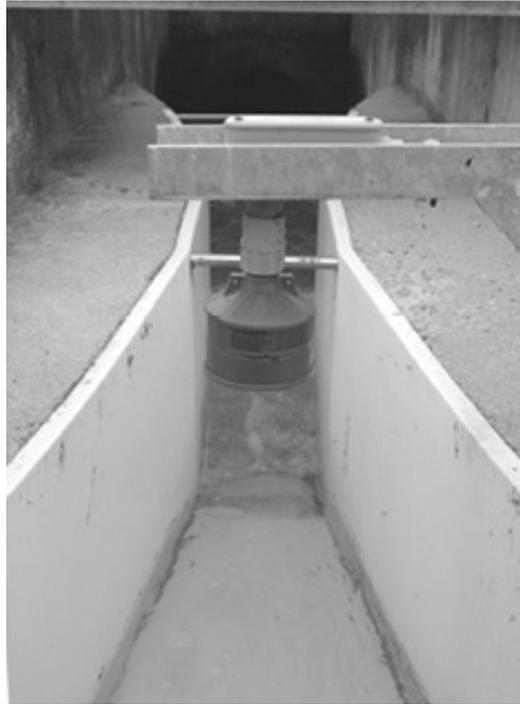
Inlet flow is often monitored using an open channel primary measuring device like a flume or weir and SITRANS LUT400, a secondary measuring device providing high accuracy level measurement using ultrasonic technology.
