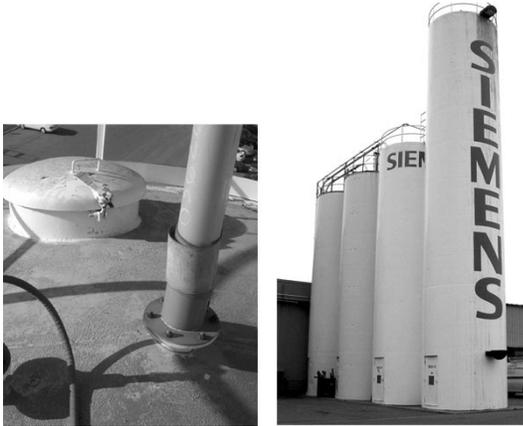
Storage vessels are typically bulk storage of liquid chemicals, hydrochloric acid, or sulfuric acid. Stored in vessels ten meters (33 ft) or less, they present no challenges to the ultrasonic system other than requiring that the wetted material of the transducer housing is compatible with the material in the vessel.
