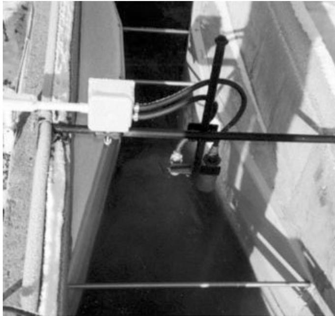
To achieve accurate flow monitoring and comply with legislation requirements, a primary measuring device combined with the LUT400 open channel monitor can be used. The LUT400 converts high accuracy ultrasonic level measurement to a flow value using known head versus flow formula or British and ISO Standards. Full data logging capabilities are available to log daily flow totals and flow rates.
