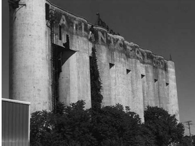
The coal silos store the coal that is burned in the kiln – the heat from the burning coal is responsible for the chemical changes of the raw feed into clinker. Ultrasonic systems monitor the level in these bins for inventory purposes.
